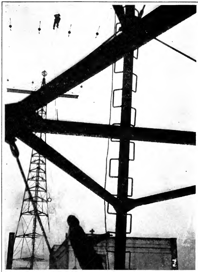
REPAIRING A BROADCAST STATION ANTENNA
